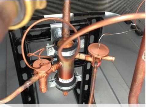
A field-installed APR Control (by Rawal Devices) for variable capacity modulation on a 5-ton R-410A roof-mounted package unit. *Image courtesy of Rawal Devices Inc.*
